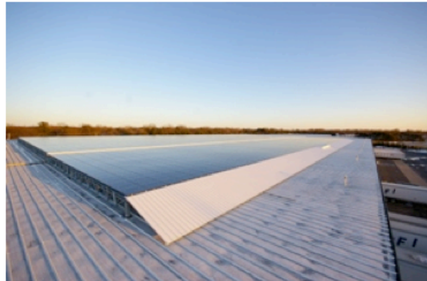
The Cherry Hill installation is the largest to date from Prot-Tech and Whitman. (Pro-Tech photo)
